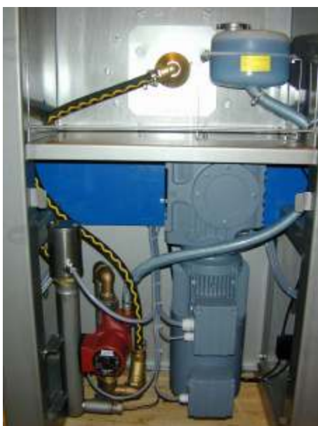
Dose VGI drive and heating system
